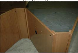
Simply use the extra 1-1/4" bronze connector bolts provided in the Adder hardware in place of the 2-1/2" connector bolts used to attach the back panel to the Adder panel. All other assembly procedures are the same.
